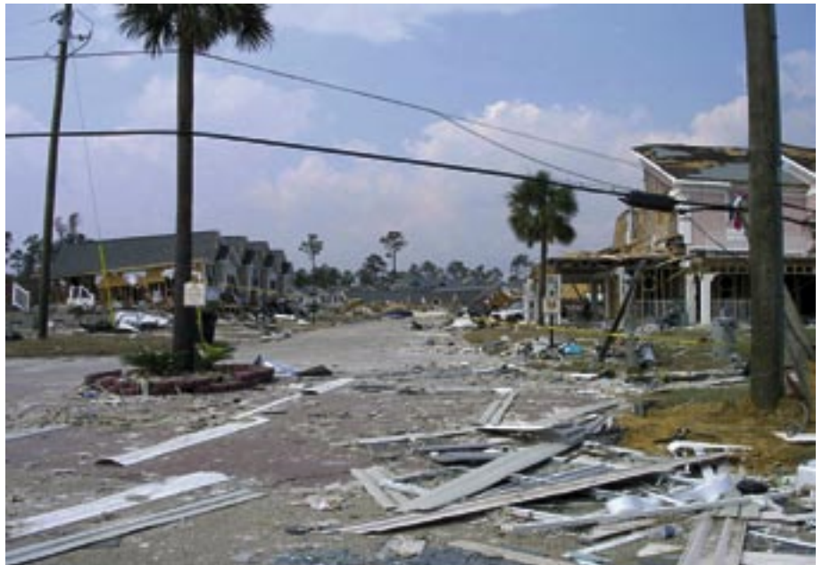
The aftermath of Hurricane Katrina in Gulfport, Mississippi, USA. ISO/TC 223 is developing standards to improve the preparedness for and response to such disasters. Photo: Rick Earls.
